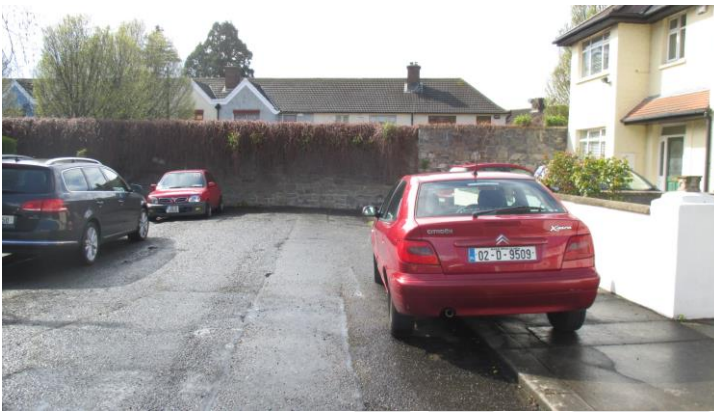
Figure 3.20: Section of existing wall to be knocked to permit access to pedestrians and cyclists.
